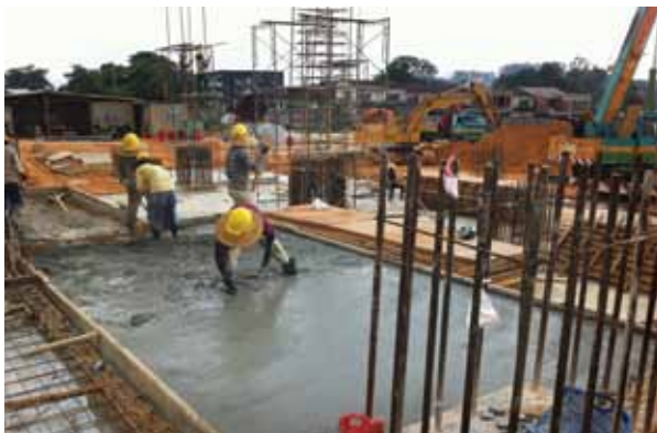
Construction in progress
